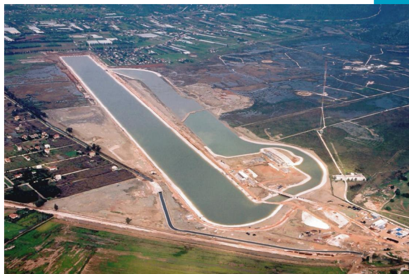
Open detention tank (multipurpose facility: BMP and water sports arena)
