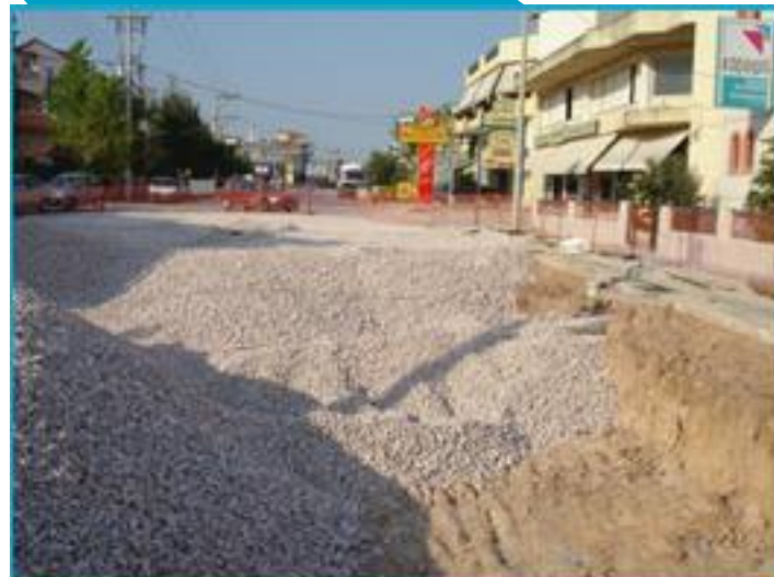
Under paving storage structures (under construction)
