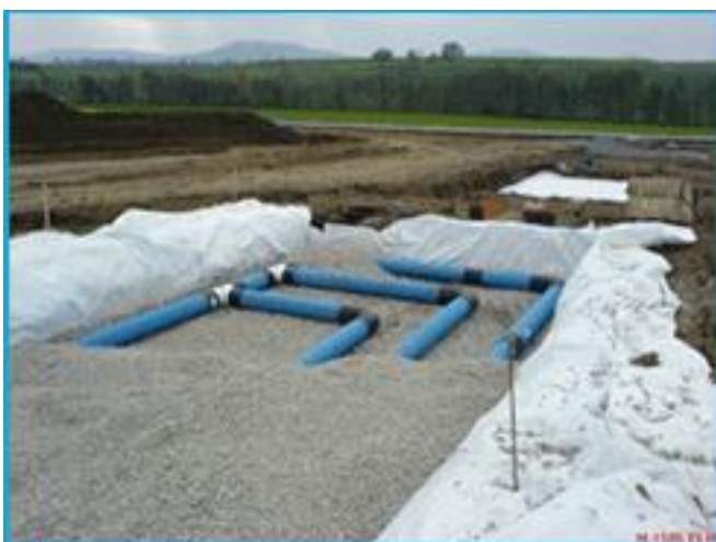
Stone filled soakaways (under construction)
