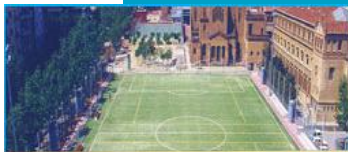
Retention concrete tank
